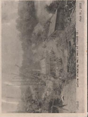
The Medina Canal Basin was under construction when this picture was taken July 31, 1913. In the center we see the great retaining wall being built using wooden forms for poured concrete.
