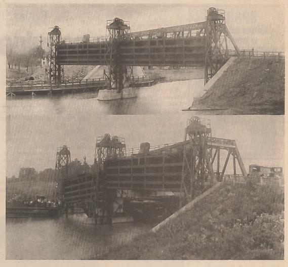
of the center tower has been partly crumpled and slightly shifted out of line, causing the gate to come down on the barge.
