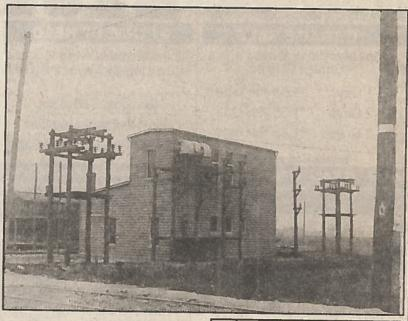
Power Co. Poles to hold the trolley power line were made of chestnut placed 110 feet apart.
