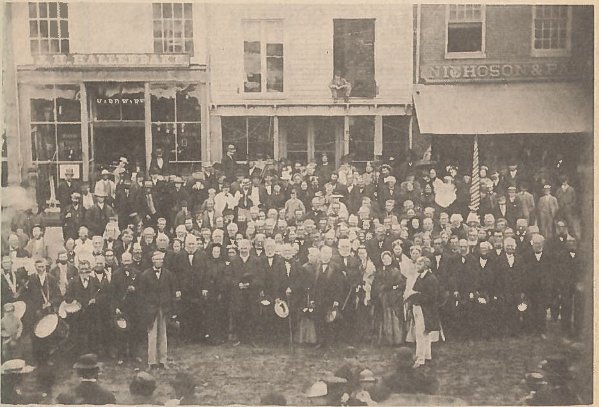
GEO. P. HOPKINS, Photographer, Albion, N. Y.
