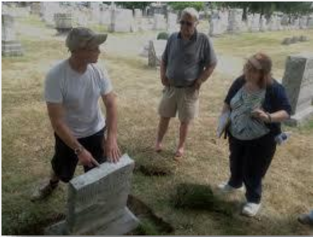
Brian Daddis demonstrates mortar repairs at a local cemetery.
