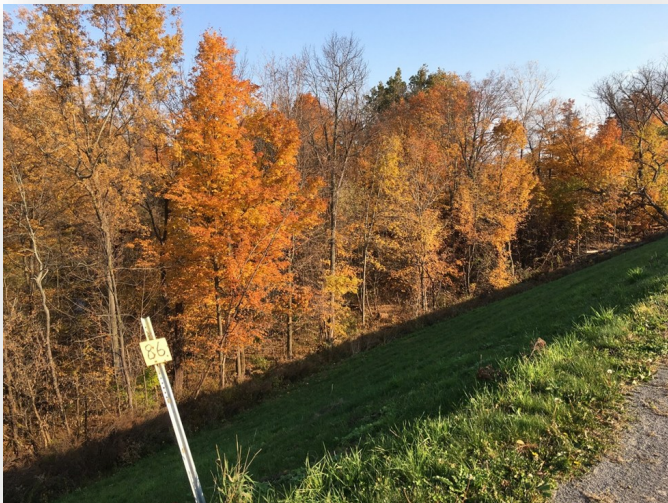
A portion of the embankment passing over Otter Creek today, known as state canal culvert #86.
