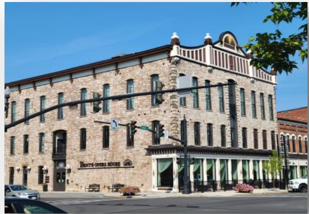
Bent's Opera House, Medina, Roger Hungerford—Talis Historic Restoration
