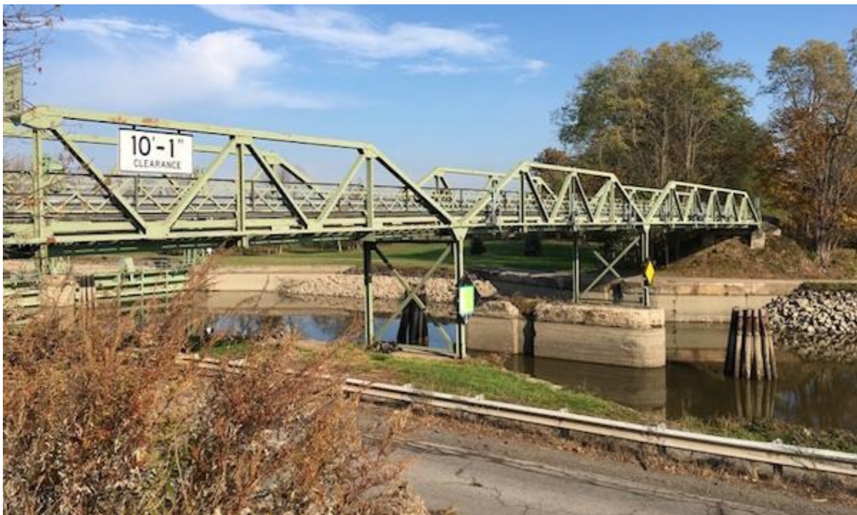
Lattin Bridge today
