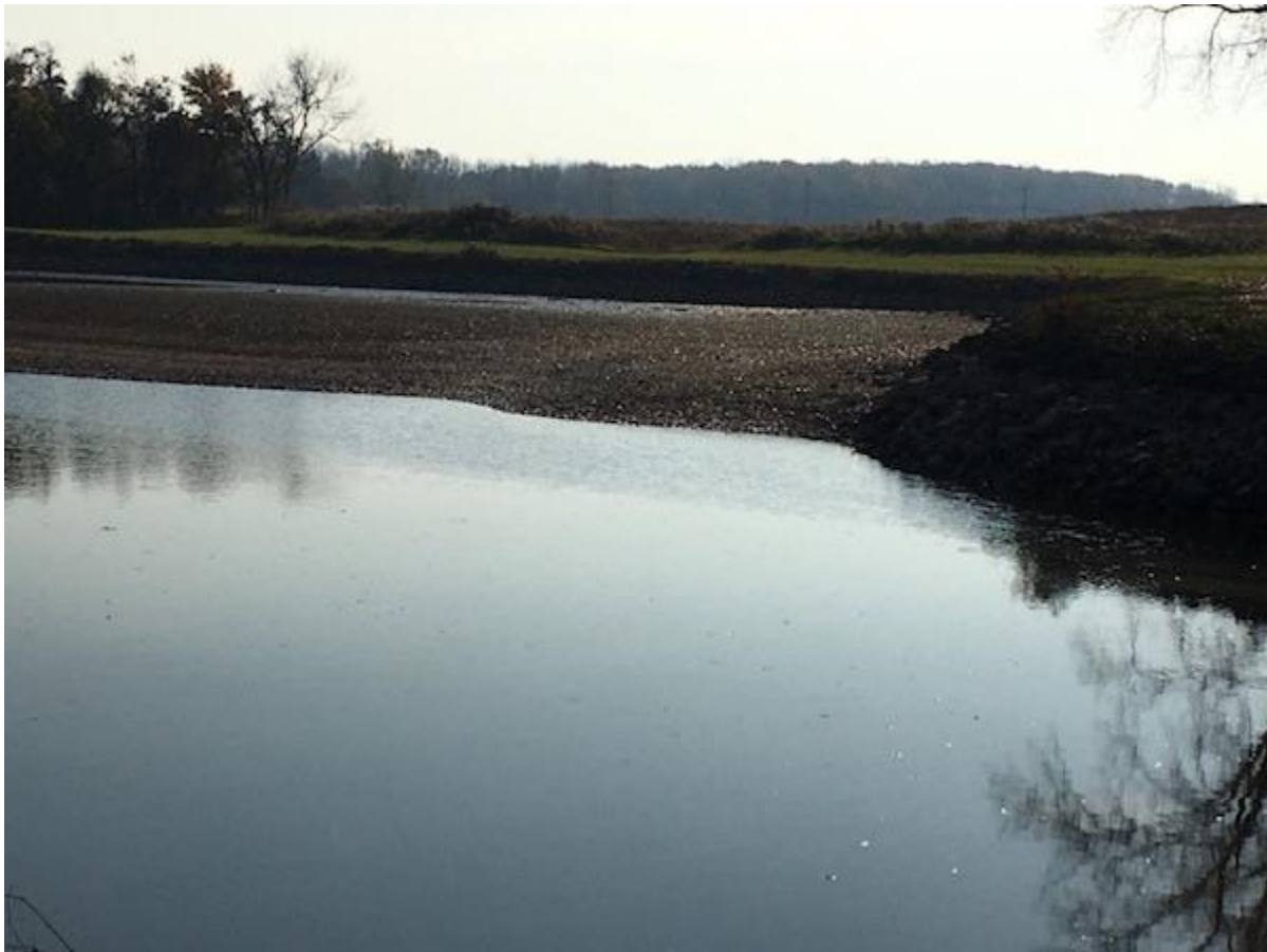
Canal Turn Basin, Town of Gaines, 2021, Canal partially drained
