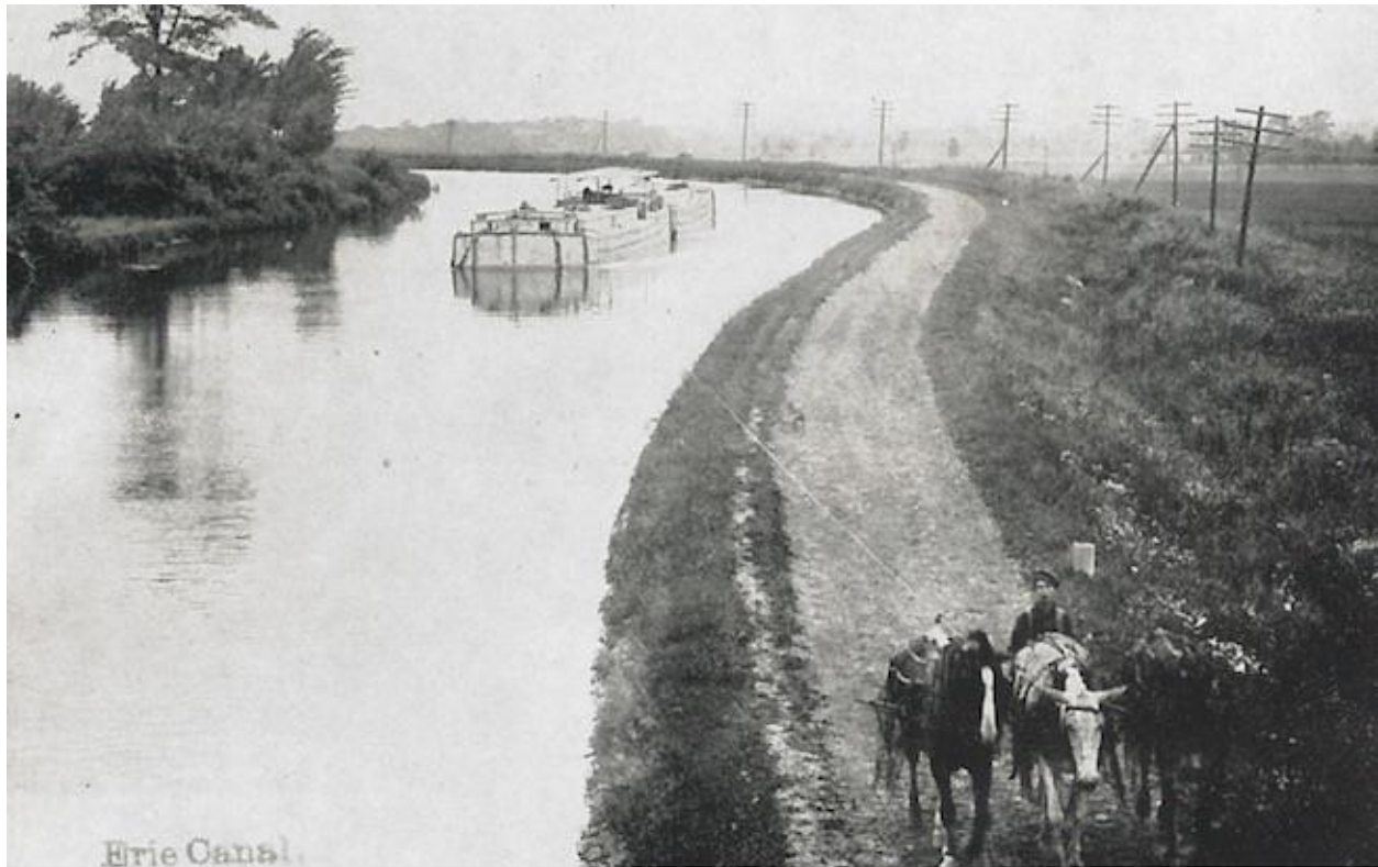
Erie Canal towpath, Gaines Basin, c. 1900 before Barge Canal expansion
