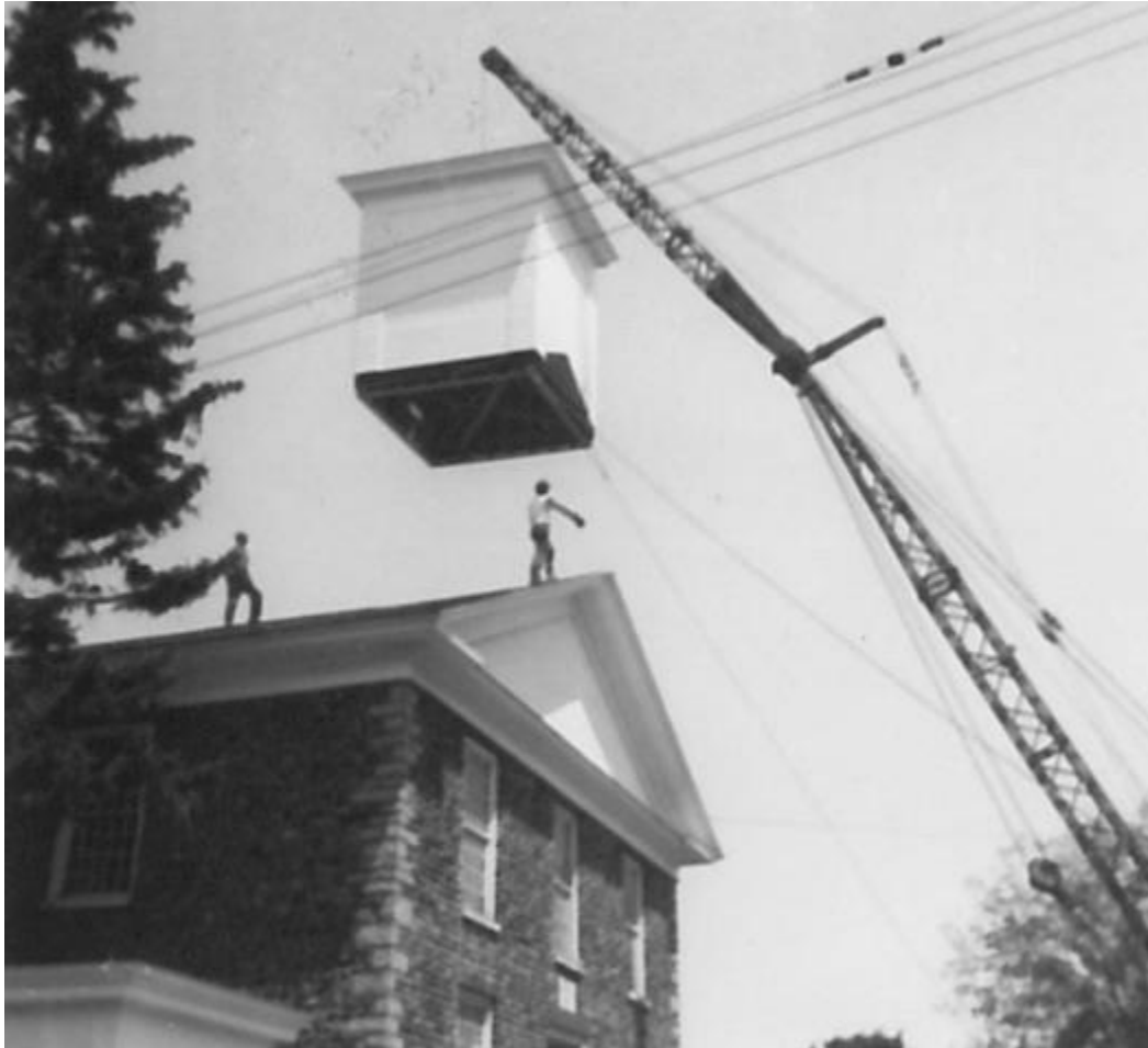
Cobblestone Church tower restoration, 1966
