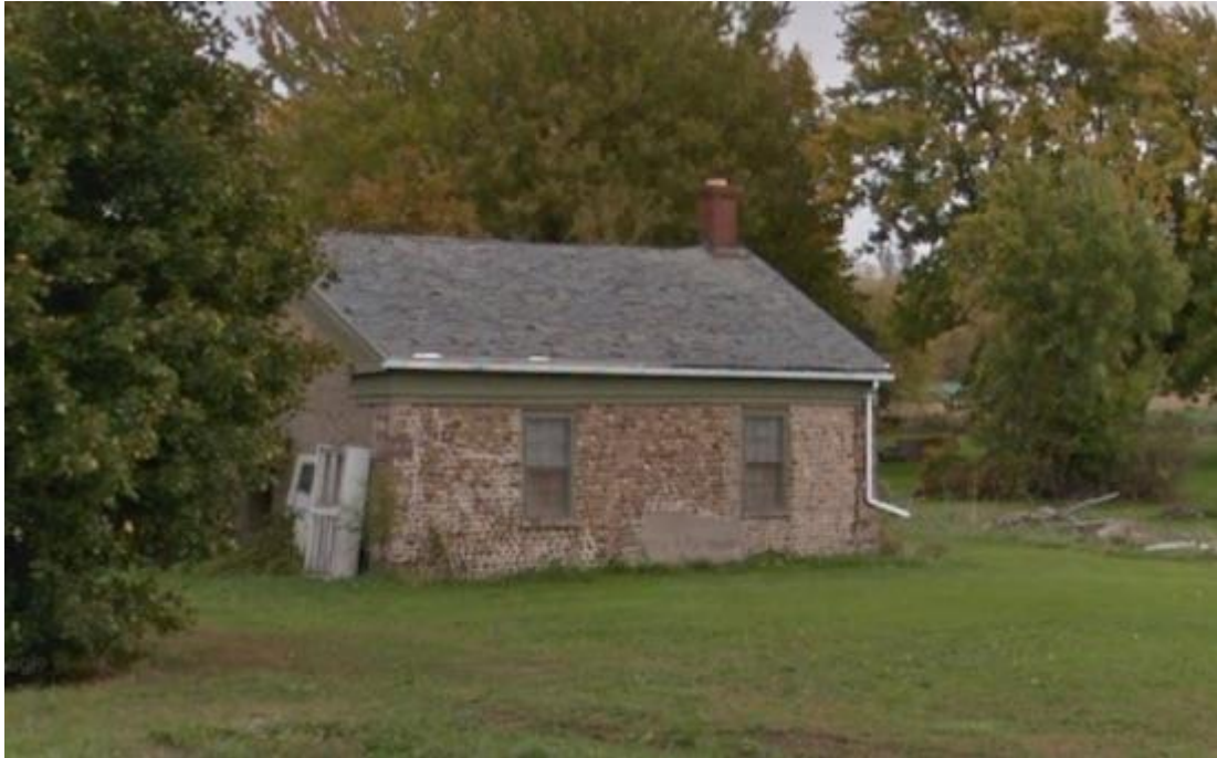
Jacqueline and Bill Bixler recently acquired the District #1 Cobblestone School and have been busy restoring it for use as a residence.
