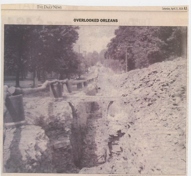
PHOTOGRAPH COURTESY OF ORLEANS COUNTY HISTORIAN'S OFFICE This image from 1908 shows a rather rocky section of East Center Street, Medina, looking west toward downtown Medina at the intersection of State Street. The work was part of an expansion of the village's sewer system.
