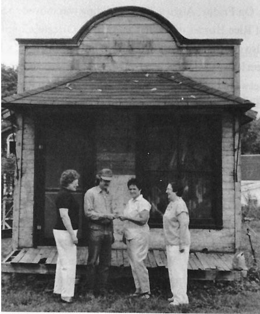
The little shop passed to the Cobblestone Society in 1987 when owner Rose Welles, notified Cobblestone Museum director C. W. Lattin that she would donate the building to the Cobblestone Museum complex. Shown above (left) is Delia Robinson, Town of Gaines Historian; C. W. Bill Lattin, Rose Welles, and Janice Thaine, Gaines Deputy Historian.
