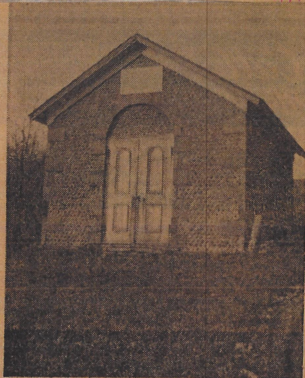
COBBLESTONE RECEIVING VAULT of the Guilderland cemetery at Osborn's Corners. The marble tablet above the door bears the inscription, "Guilderland Cemetery 1872 Receiving Vault." The cemetery itself is much older than the vault. It is also known as the Dutch Reformed cemetery, being located on the original lease of 43\frac{3}{4} acres from "the proprietor of the Manor of Rensselaerwyck, Stephen Van Rensselaer, Esq., to the Minister, Elders, and Deacons of the Reformed Protestant Dutch Church of the Hilleberg." The lease was dated October 25th, 1794.
